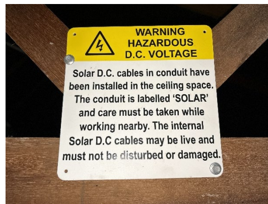
Figure 1: A compliant label installed adjacent to the access point of an accessible roof space.
