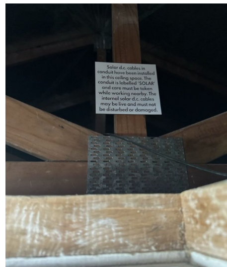
Figure 3: Non-compliant: the label does not contain the WARNING: HAZARDOUS d.c. VOLTAGE portion of the label.
